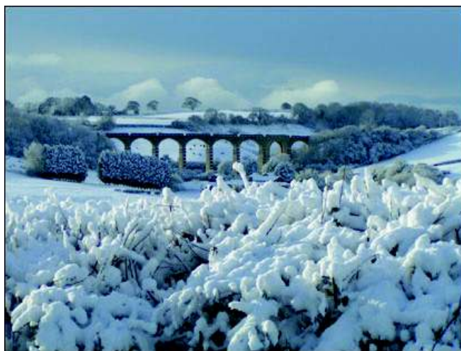
Cannington Viaduct, near Uplyme, East Devon on the morning of Friday 25 November 2005 (Photograph courtesy of Joss Kent)
